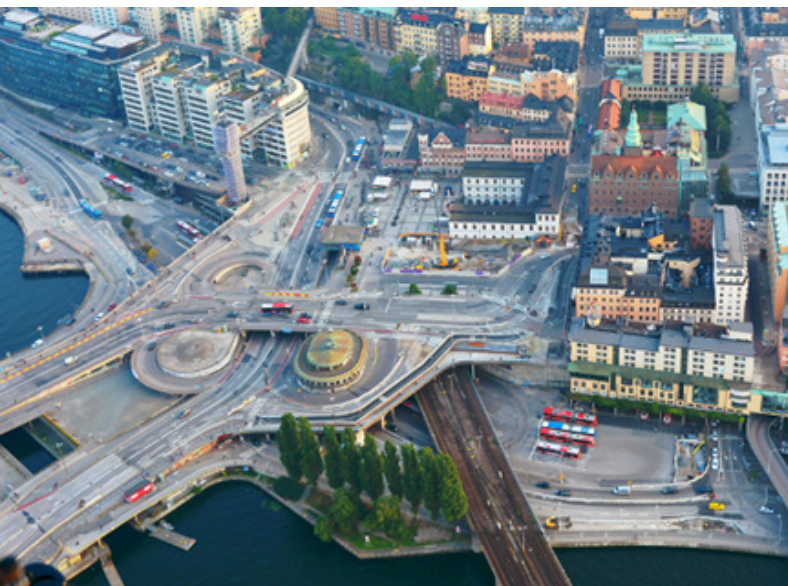
Slussen was given its name in 1935, in connection with the inauguration of a new traffic interchange and a new lock. The Slussen Carousel was Europe's first cloverleaf interchange in an urban setting and created a new traffic hub in central Stockholm. Photo: Johan Fredriksson
